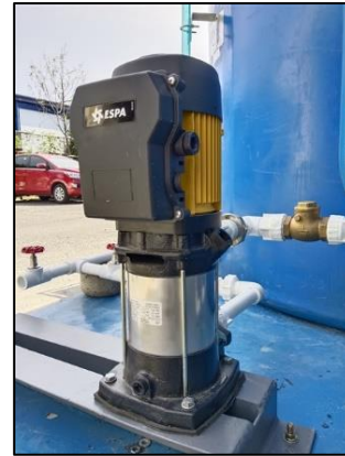
Figure 11. RO Reject Water Distribution Pump
