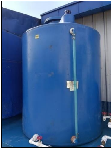
Figure 10. RO Reject Water Harvesting Tank
