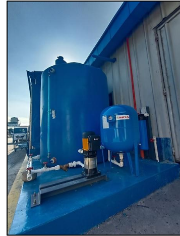
Figure 7. RO Reject Water Harvesting System
