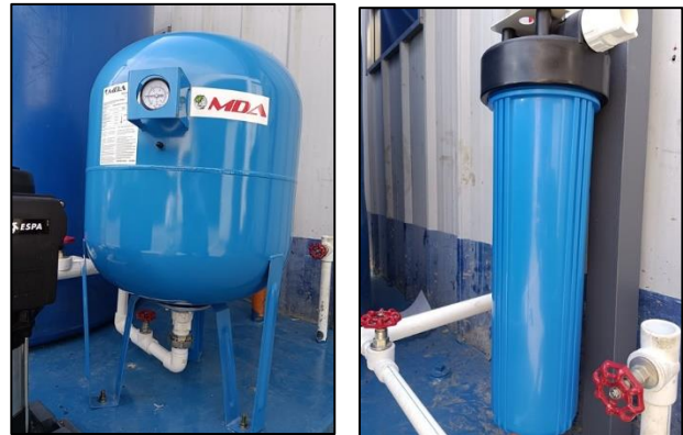
Figure 12. Pressurized Tank and In-line Water Filter
