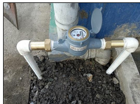
Figure 13. Discharge Water Meter
